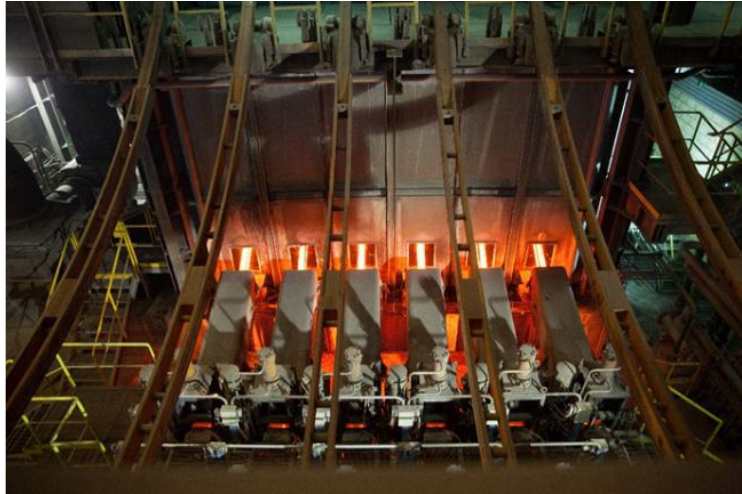
Figure 4: Continuous casting machine.
